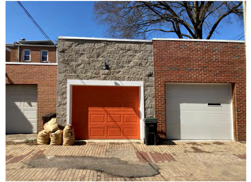
GARAGES ACROSS ALLEY
