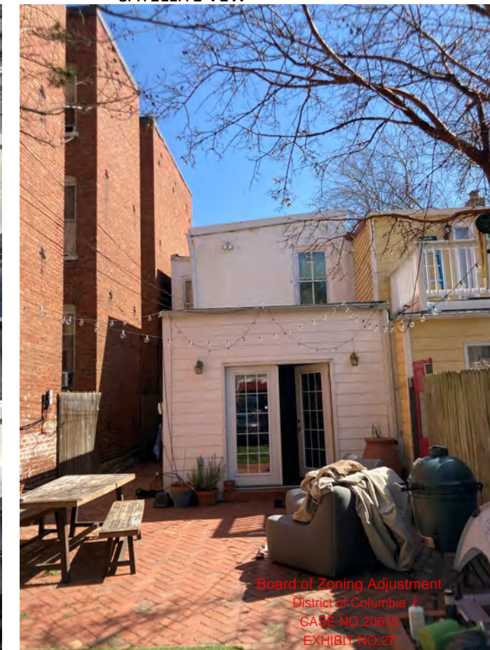
EXISTING REAR FACADE
