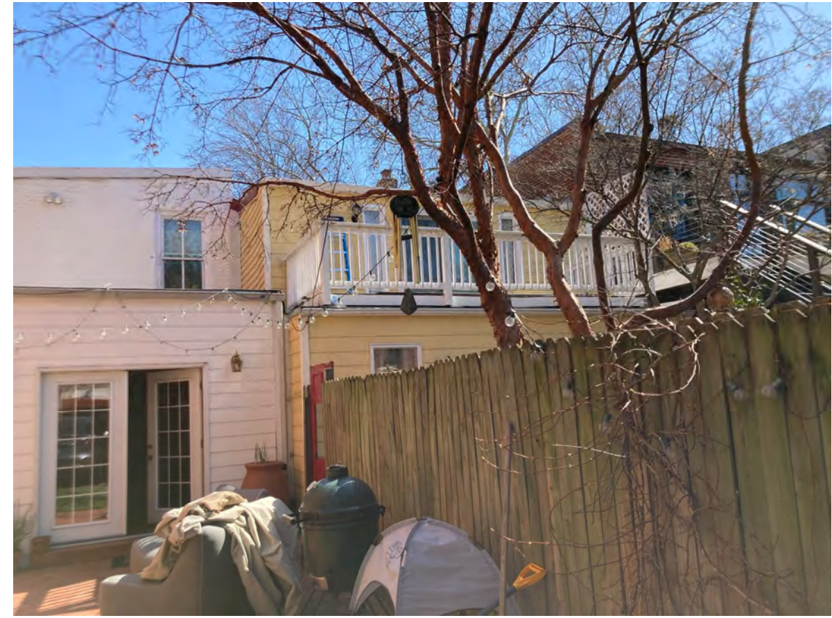
VIEW TO THE SOUTH
